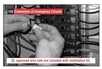
NOTE: Circuits to be moved must be protected by same size breaker. For example, a 15 amp 120V circuit in emergency load center will replace a 15 amp 120V circuit in main panel.
